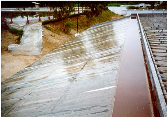
Fig. 3 Distribution channel and flat plate collector
