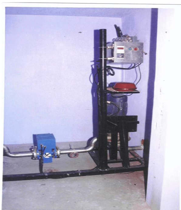
Picture 2 – Flow meter installation
