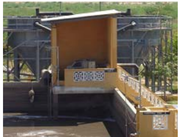
Picture 6 – Rotary screen & pre-settlers
