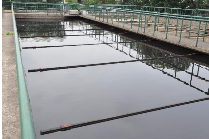
Figure 7: Effluent treatment plant; Shanghai, China
